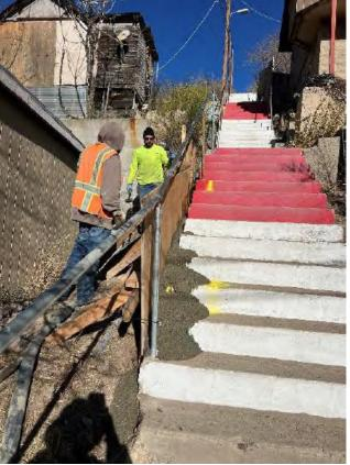
Work Scope: Repairing or replacing existing damaged concrete on the stairs, landings, and ramps, replacement of existing retaining wall, extension of retaining wall, and addition of handrails.
