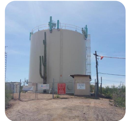
Mammoth Water Tank #1 Rehabilitation.
