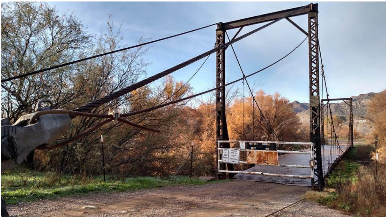
The Rafter Six Ranch Bridge over the Gila River. Photo Courtesy of Officer Curt Holloway.
