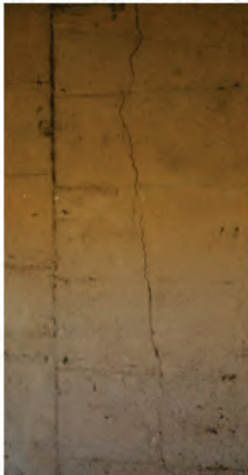
Typical pier vertical cracks
