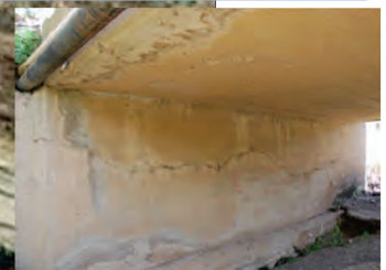
North abutment, Wide horizontal crack
