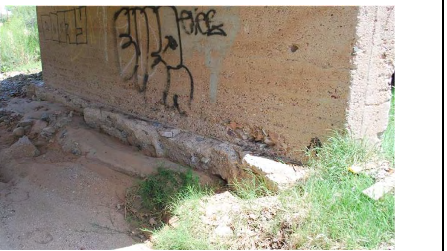
EXISTING PIER FOOTING/CAP
