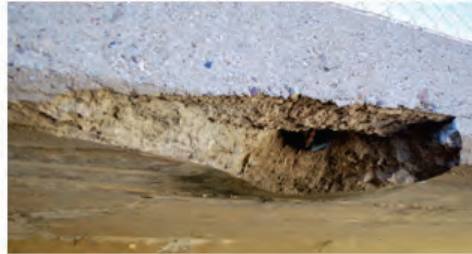
Sidewalk overhang spall, east edge, south end
