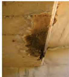
Delaminating Drainage Retrofit, North end, east face
