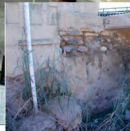
South abutment wall spall
