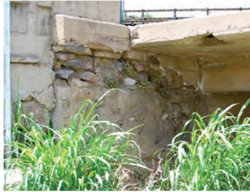
South abutment wall spall
