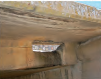
Delaminating Drainage Retrofit, North end, east face
