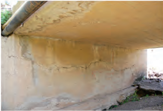
Typical pier vertical cracks
