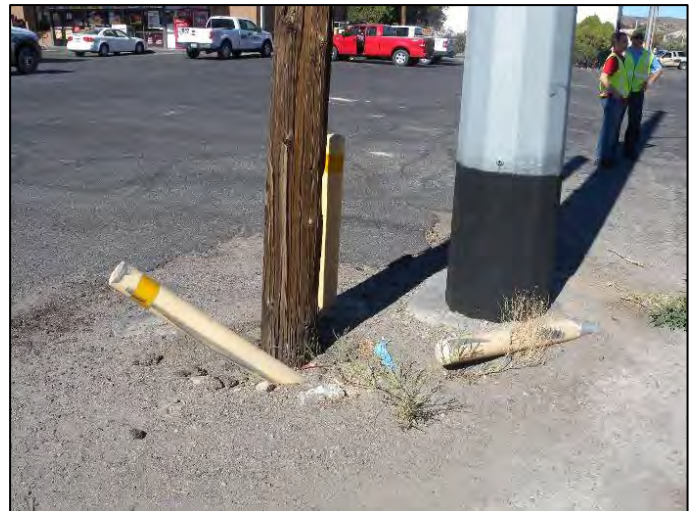
Figure 9: Bollards and Pole on Southwest Corner of Circle K Lot Have Been Struck by Vehicles
