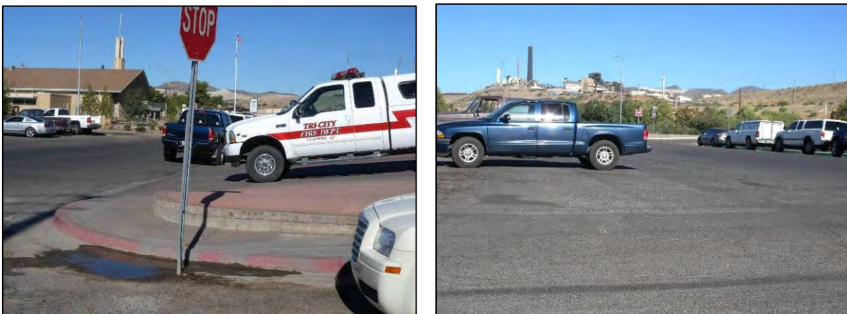
Figure 11: Sight Obstructions at the Broadway Street/El Camino Street Intersection Created by Parked Vehicles
