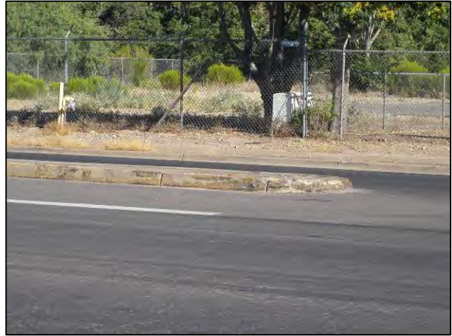
Figure 13: Median Bullnose Has Been Struck and Run Over Numerous Times
