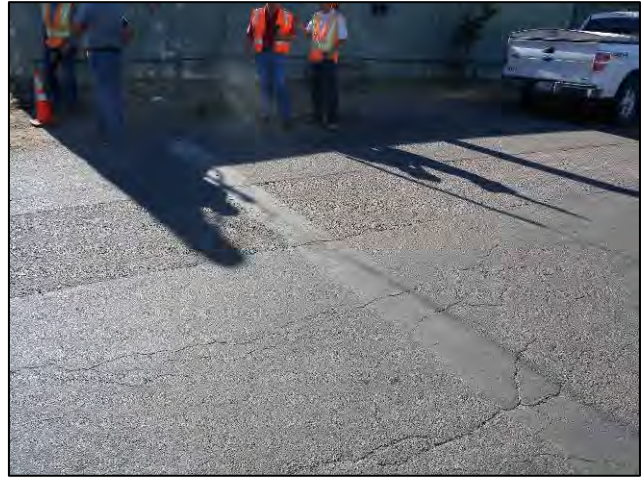
Figure 15: Faded Centerlines and Stop Bars
