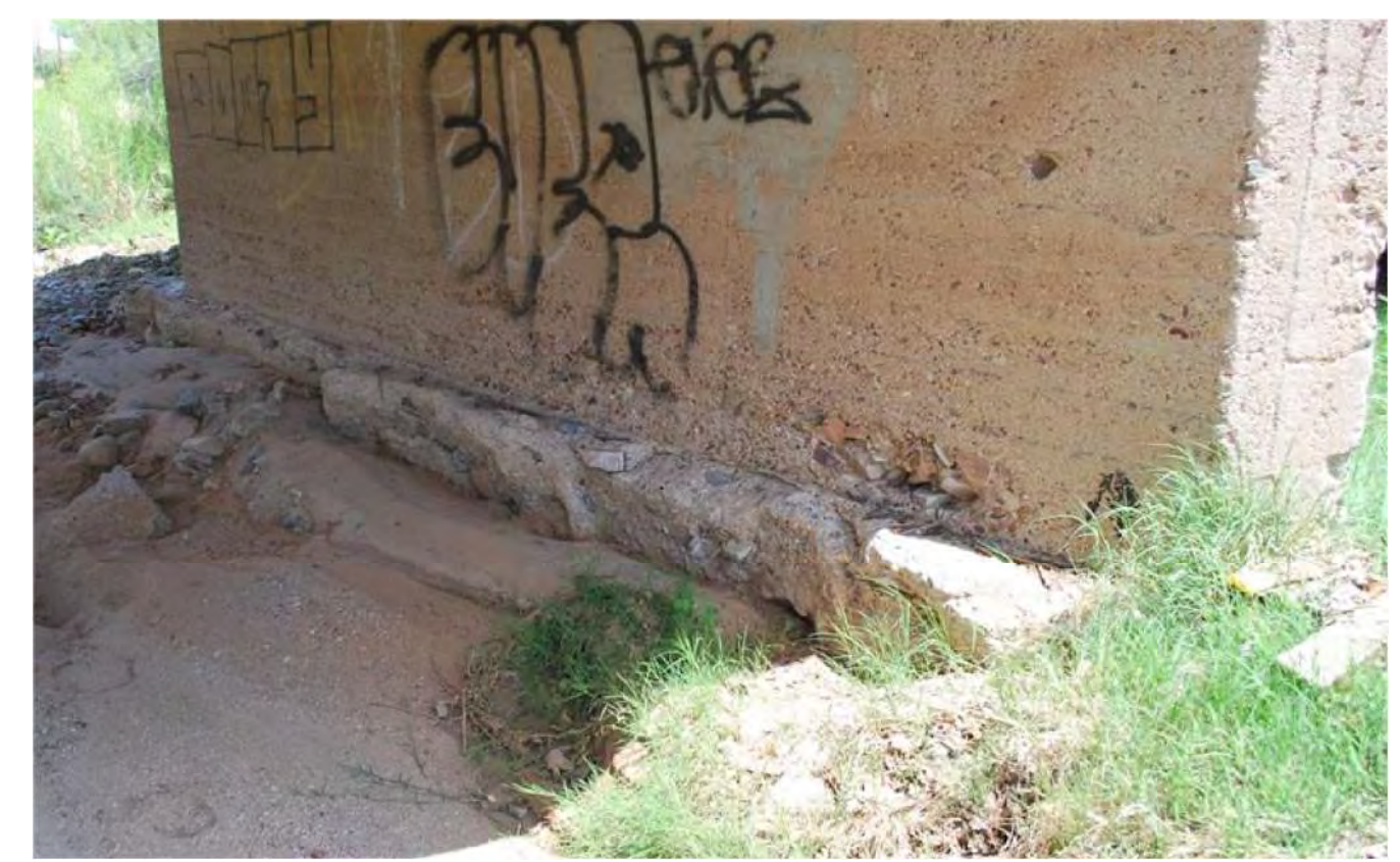
EXISTING PIER FOOTING/CAP
