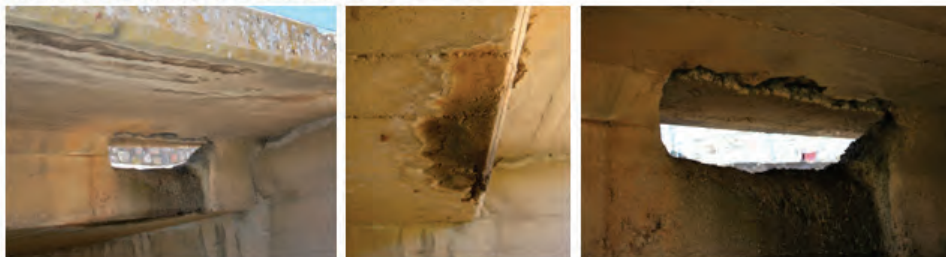
Delaminating Drainage Retrofit, North end, east face
