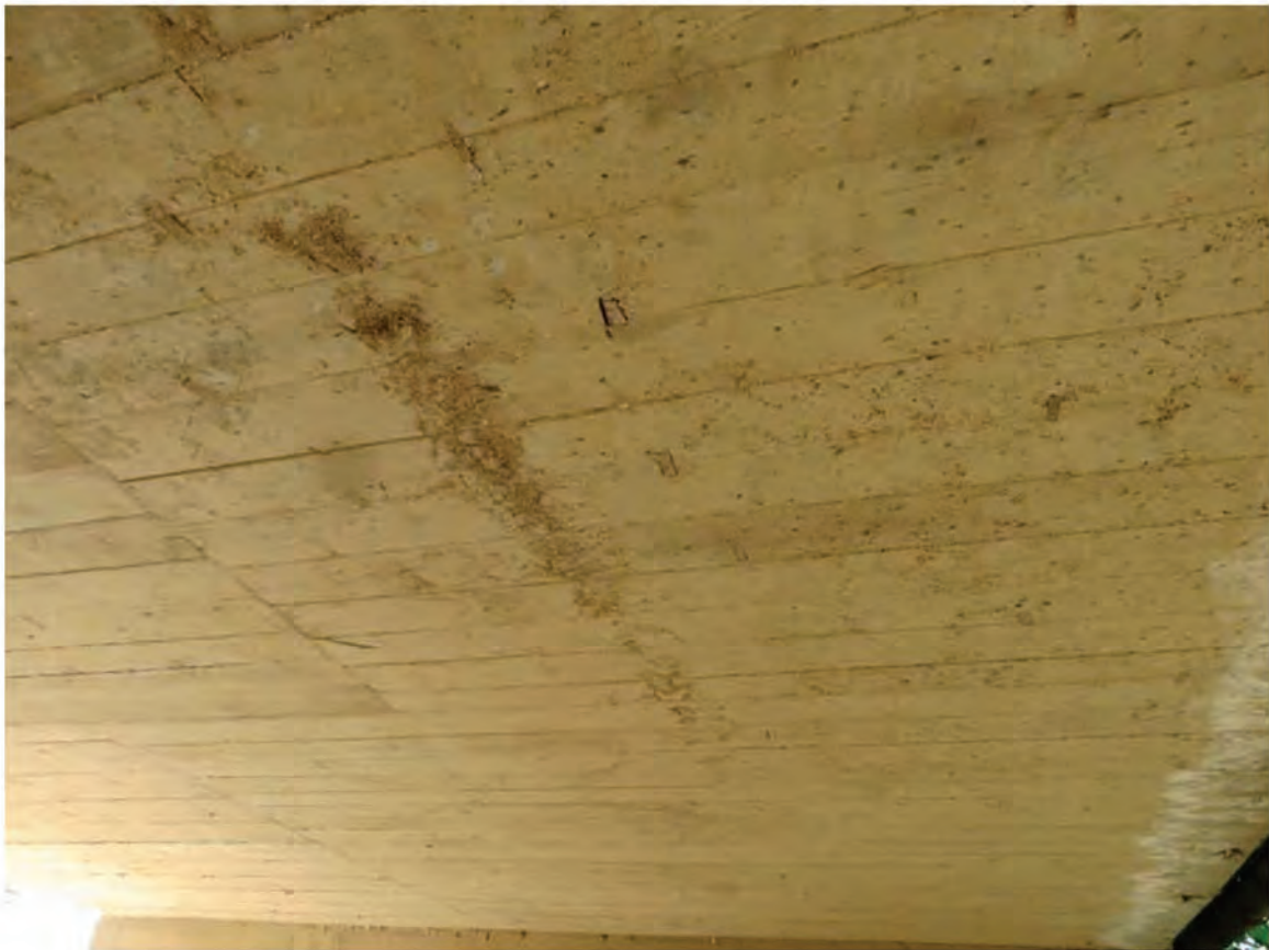
Photo No.: 4 File Name: 0971017d.jpg Descriptions: Deck bottom
