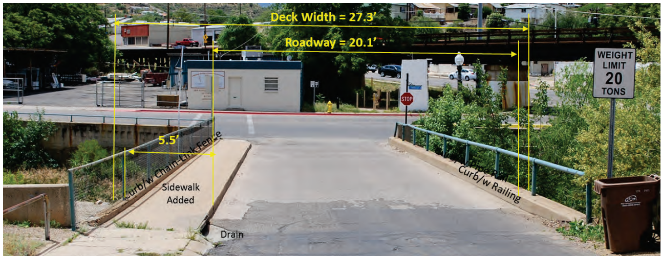
Figure 3: BRIDGE GEOMETRICS (LOOKING SOUTH)
