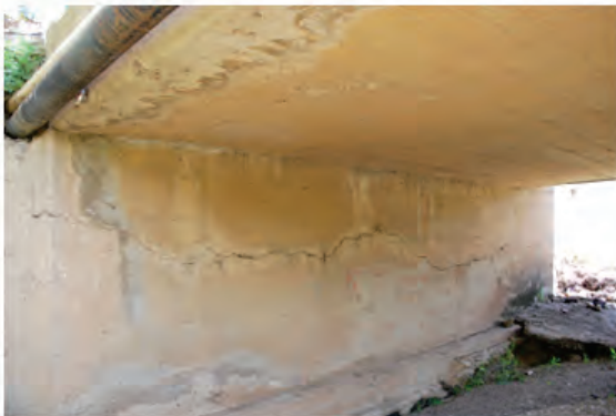
Typical pier vertical cracks
