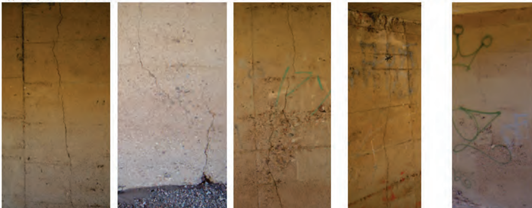
Typical pier vertical cracks
