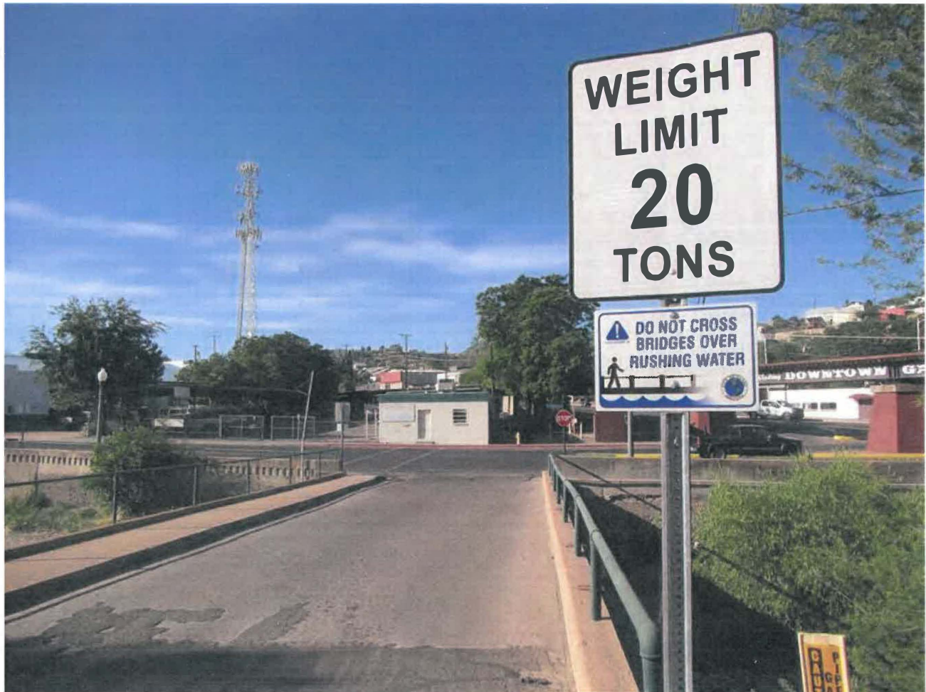
File Name : 09710-2022-05-06-Photo-06.JPG Description : Load posting sign at north approach
